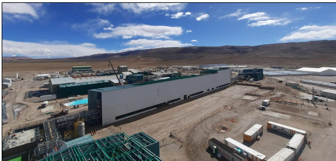
Figure 14-7. Photograph of Project Fenix Current Facility First Expansion, January 2023
