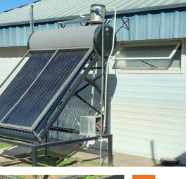
Bottom image: Solar hot water heater for domestic water use
